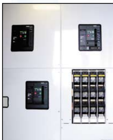
L.V. distribution panel closed design
