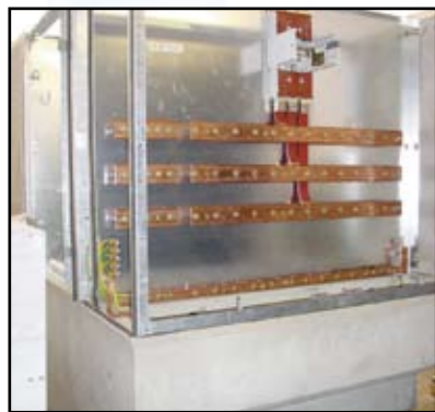
Foundation and metallic frame
